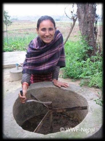
The methane produced in the digester of a biogas plant when naturally occurring bacteria acts on the mixture of dung, excreta and water. The gas is used for lighting and cooking.
